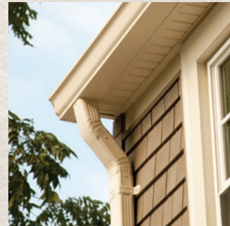
Rainware, Fascia, Soffit
